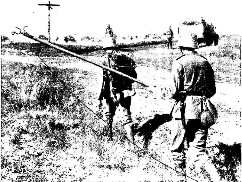
Figure 145.—Reeling out field wire.
