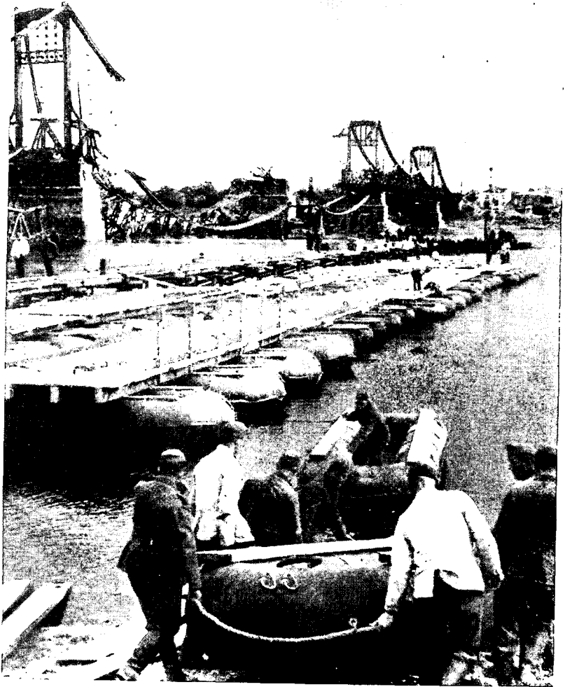
Figure 123.—Ponton bridge under construction.
